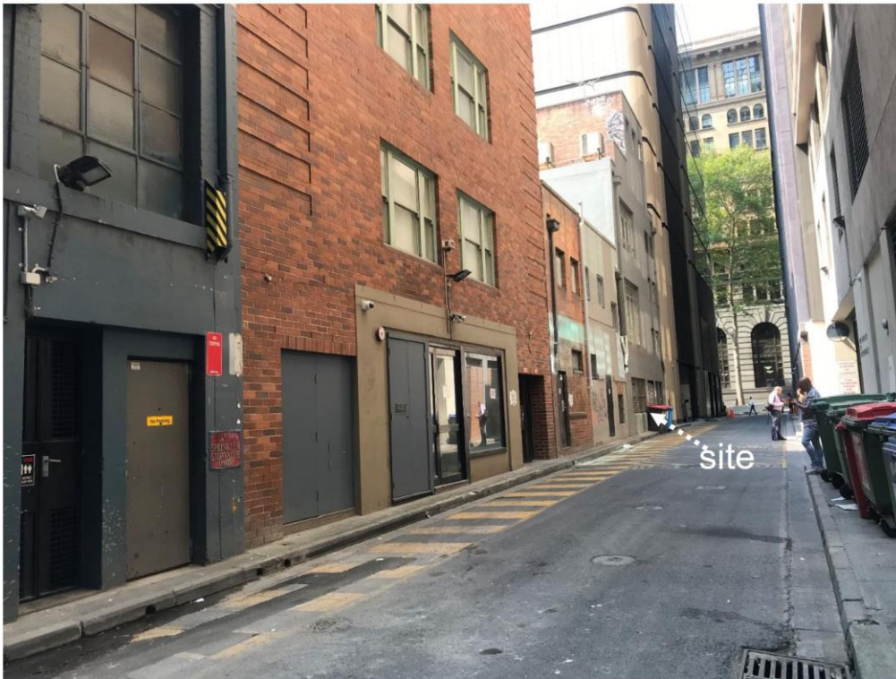
Figure 15: Looking south along Wynyard Lane
