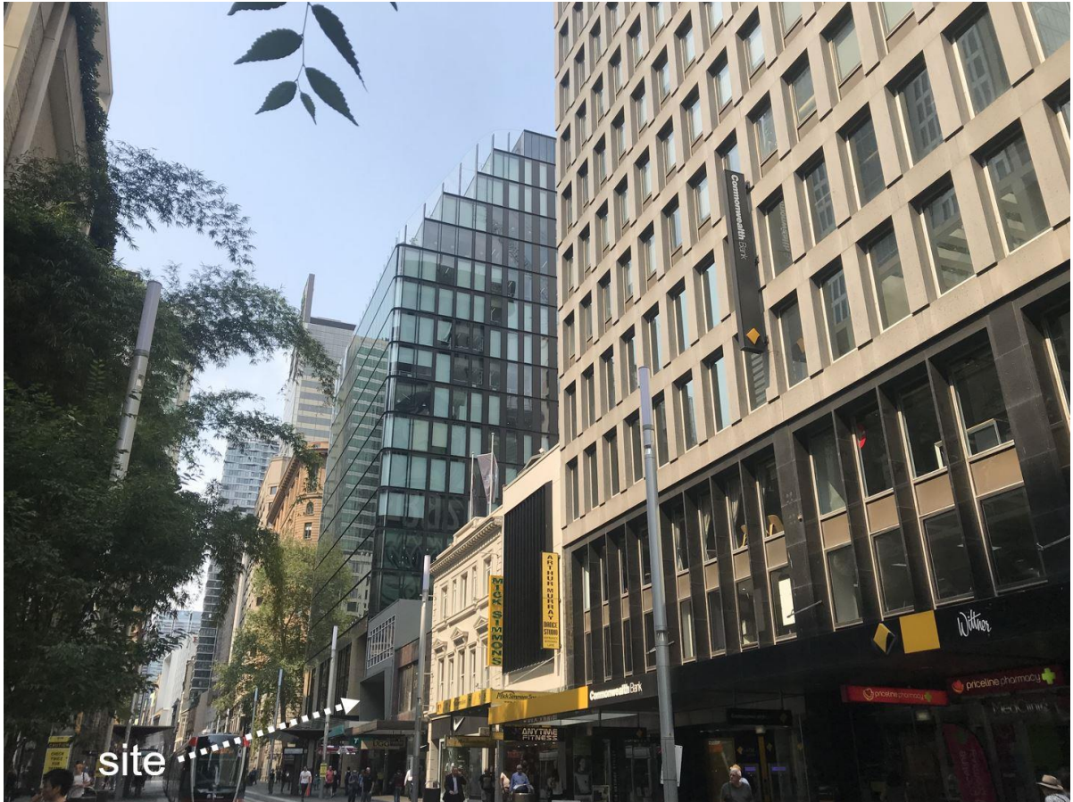
Figure 5: Site viewed from George Street, facing south-west
