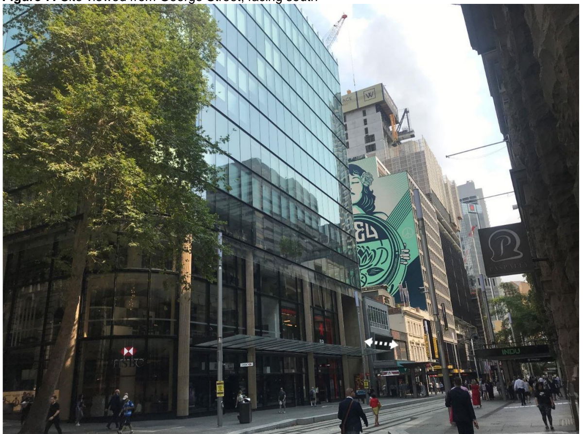
Figure 8: Site viewed from the corner of George Street and Martin Place
