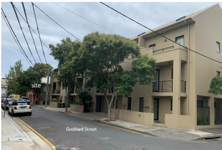
Figure 6: 2 storey townhouses adjoining the northern boundary of the site (1A-1F Goddard Street).
