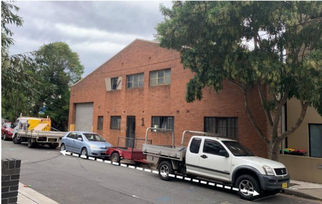
Figure 3: Site viewed from Goddard Street, looking south-west.
