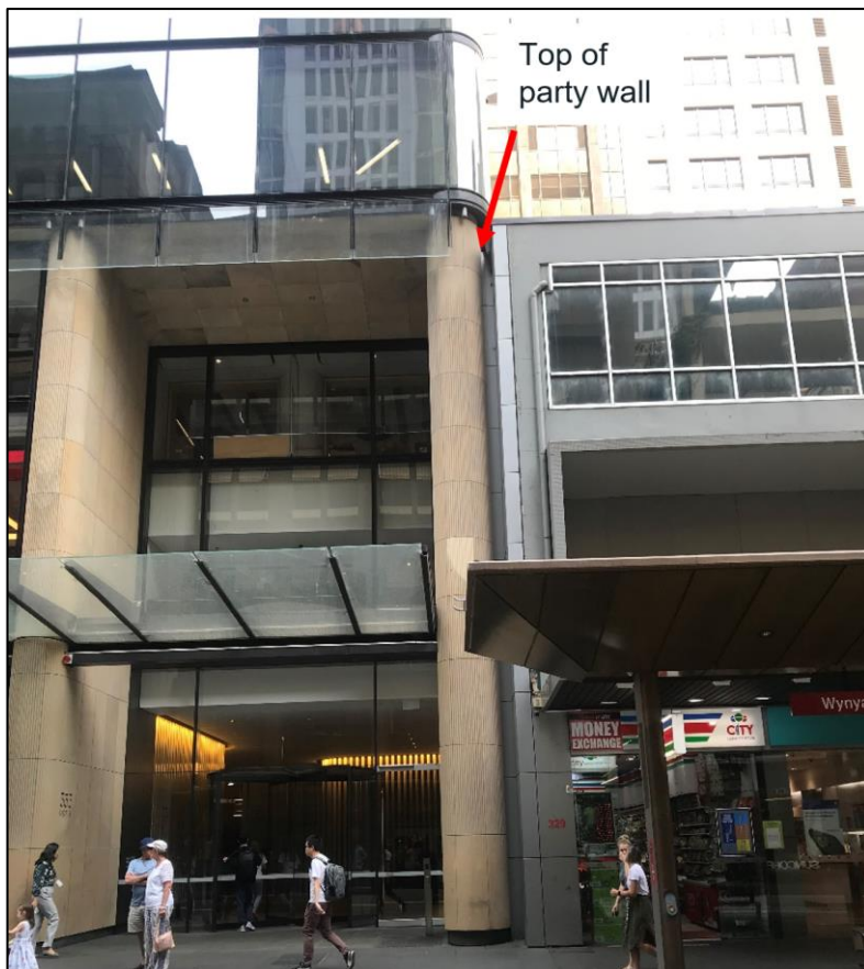
Figure 39: View of existing party wall from George Street, with top of party wall indicated
