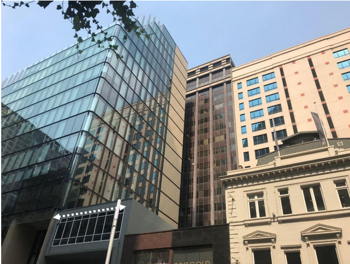
Figure 11: Site viewed from George Street, facing west
